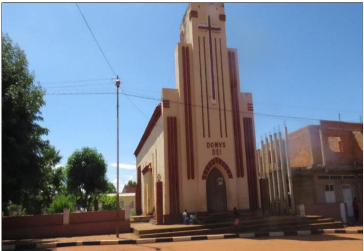
Figure 4-37: Front of the Vila parish church
