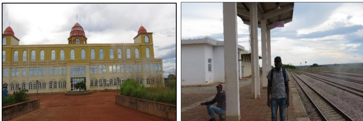
Figure 4-51: CFM station at Jamba
